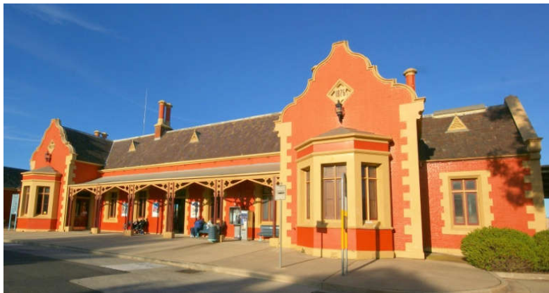
Railway Station Bathurst
